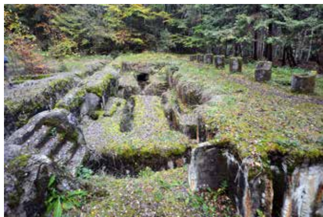
The complex at Osowka nicknamed the Power Station or the Gymnasium. It certainly seems to have been designed for heavy plant. A number of underground chambers can be accessed. Photo Chris Rayner
